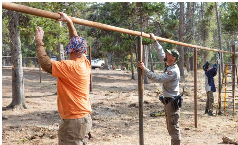
Yellowstone National Park: Canyon Corral volunteer project: tacking posts into place. Photo by National Park Service/Jacob W. Frank, 2020, public domain. Cropped.
